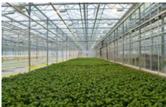
Glasshouse Operation Christchurch, Auckland
